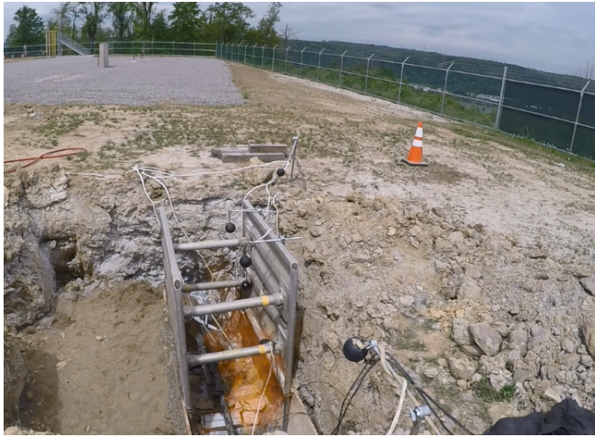
6' shored excavation with sensors in
